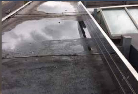
Pooling rain water on existing roof
