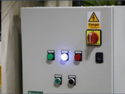
One of 7 new panels
